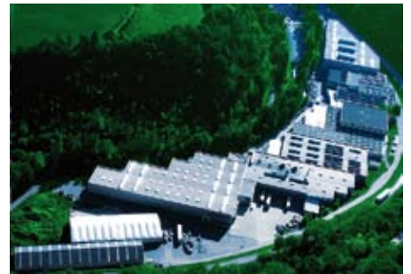
Bieringen, axial fan production in Bieringen / Germany
