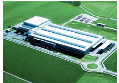
Waldenburg, centrifugal fan production in Waldenburg / Germany
